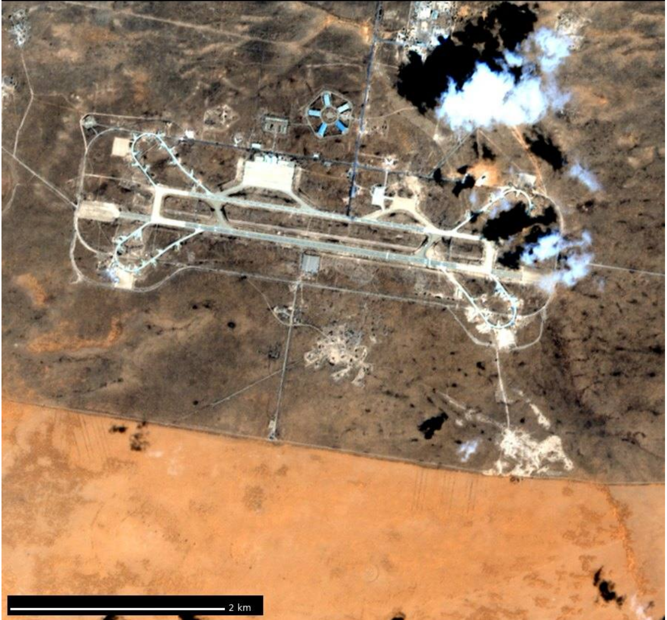
Plate B10 — Al-Watiya runway and aprons — close-up, 6 Jul 2020.
